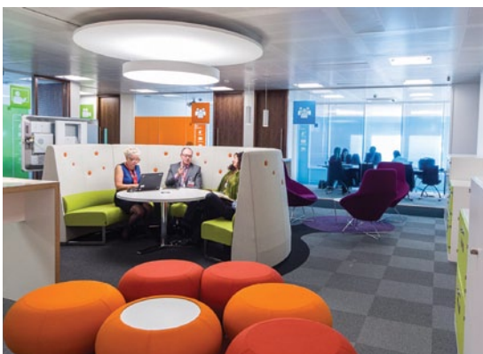
Acoustic ceiling islands to suite with the lighting and furniture
